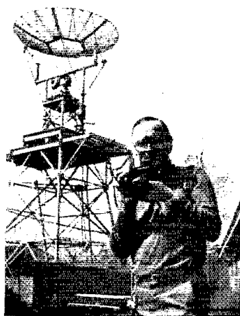
TA Paul Wilson, W4HHK, stands before his towering 18-ft dish antenna.
