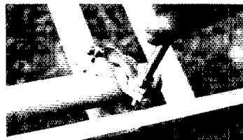
U bolts are used to clamp the lower end of the mast to one of the upper rungs of the ladder.
